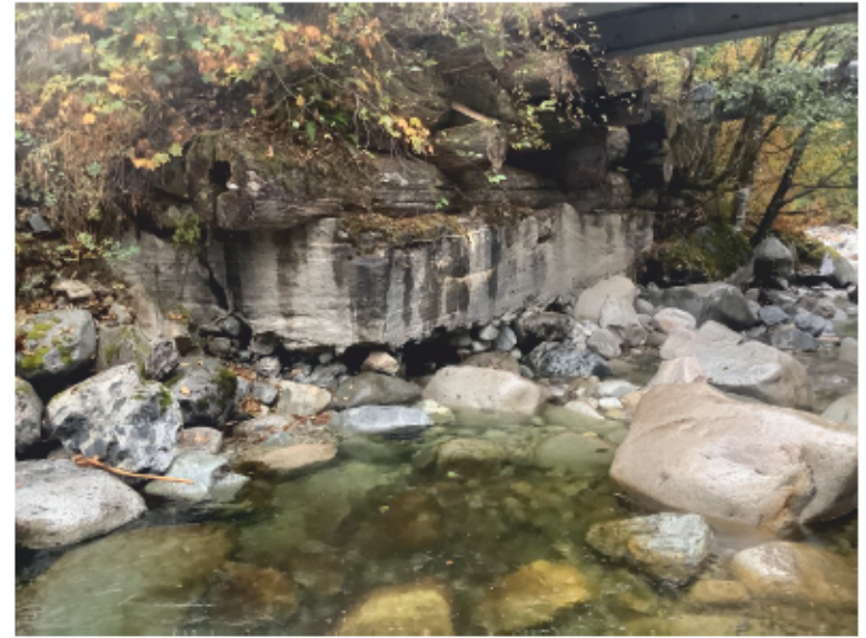
Left Bank Abutment when facing downstream
