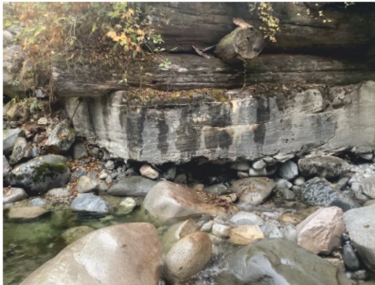
Left Bank Abutment when facing downstream
