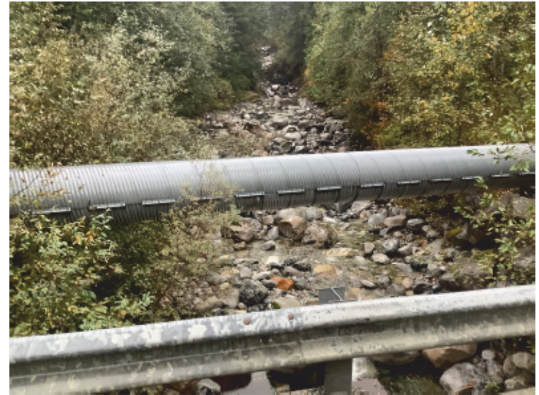
Upstream from Crossing
