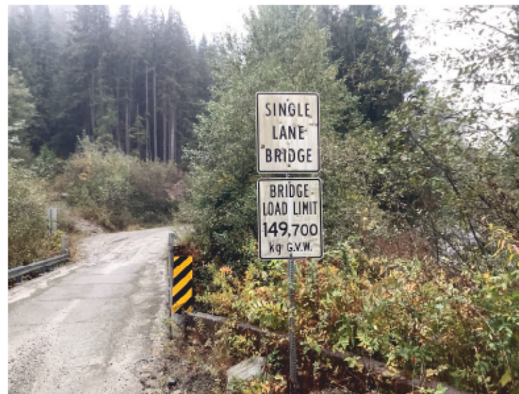
Load Rating Sign
