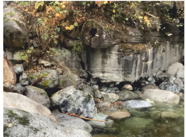
Left Bank Abutment when facing downstream
