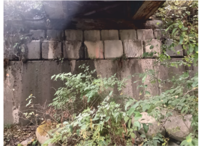
Right Bank Abutment when facing downstream
