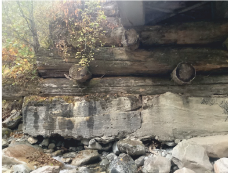
Left Bank Abutment when facing downstream
